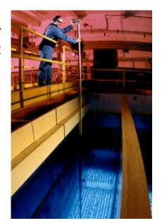
The water around the cesium and strontium capsules in the Waste Encapsulation and Storage Facility pools glows a color of blue. The effect is known as the Cherenkov Glow, as the radioactive cesium and strontium decay and lose their radioactivity to become stable atoms.
